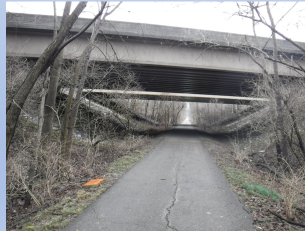
Lost Bridge Trail at I-55/I-72
